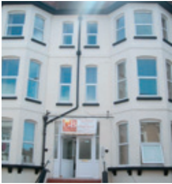
14-16 ATHELSTAN ROAD, CLIFTONVILLE
