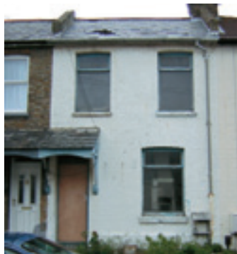
WINCHELSEA TERRACE, DOVER - BEFORE
