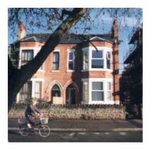
A 4-bed semi detached house built in about 1895. This house is the largest of the six case studies. It was comprehensively refurbished in 2005. The property is the architect Gil Schalom's own home. An extension was built to the rear. The side and rear elevations of the house were externally insulated and rendered. Other walls were insulated internally using dry-lining plasterboard. The roof was also highly insulated and many other sustainable features have been added.
